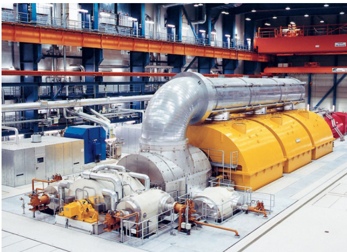
Gambar 2.6. Generator sinkron tipikal
