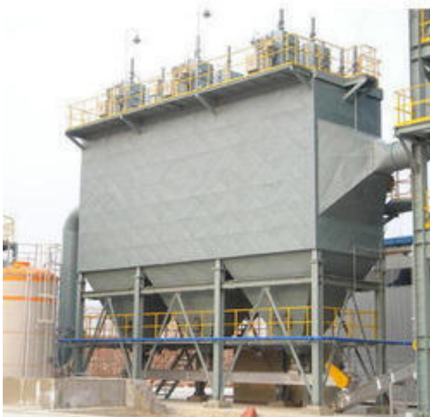
Gambar 2.12 Penangkapan abu ( electrostatic precipitator )
